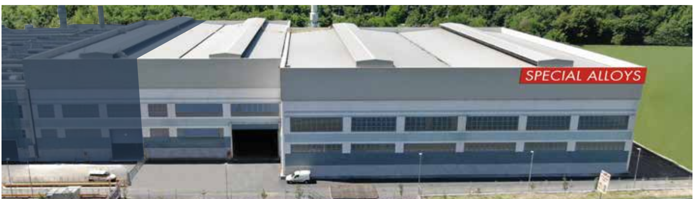
Special Alloys production plant dedicated to primary foundry alloys from recycling
