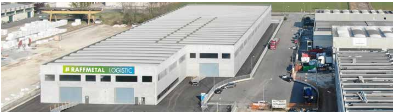
Nuvolera plant dedicated to final product storage
